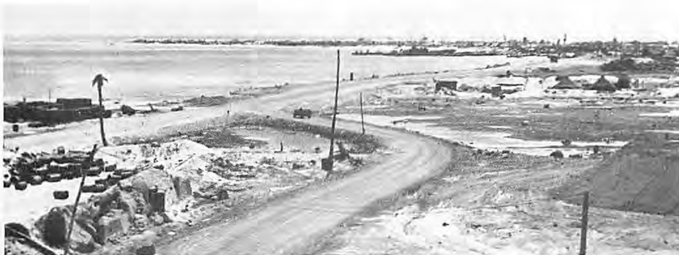
A new base takes shape: March, 1944 view shows Namur in foreground, Roi in the distance.
