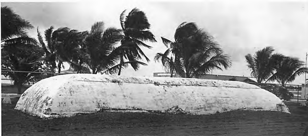
Bomb shelter in present-day fuel farm.
