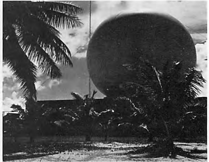
TTR-4. Constructed in 1960, the TTR-4 is one of the best known landmarks on the Island.
