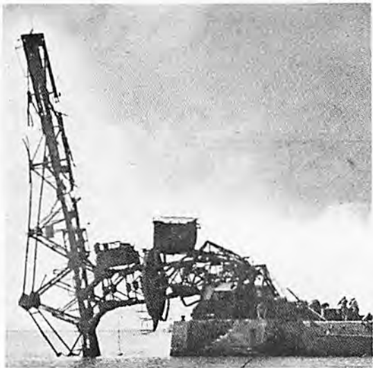
Wrecked Japanese crane, Yokohama Pier. A U.S. destroyer accidentally hit the crane with its final salvo, thereby ruining American plans to use it.
