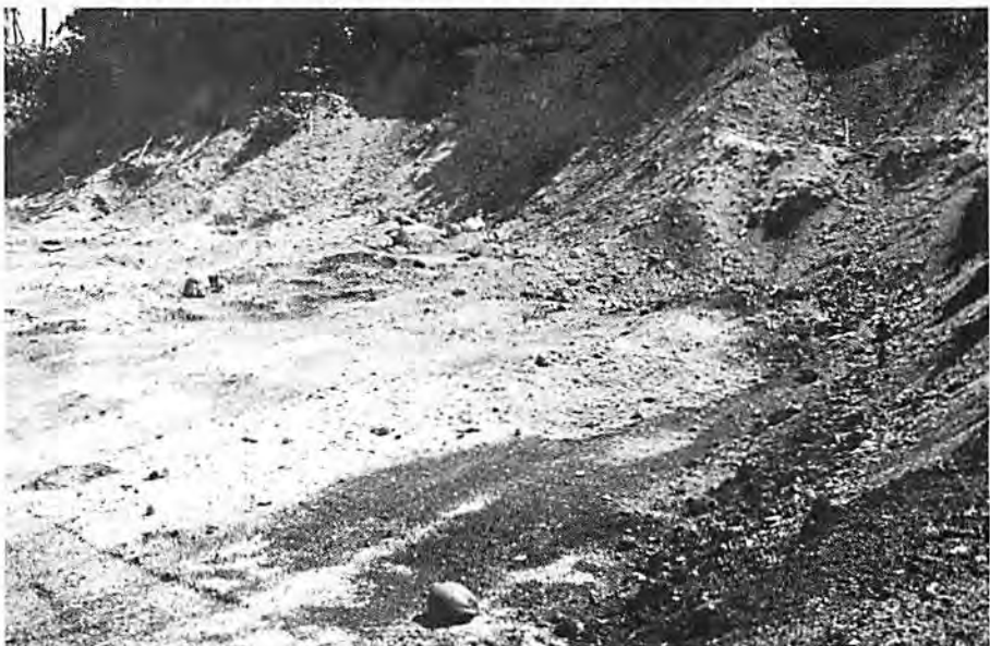
The same area today. Note the charred soil [at right] still evident thirty years later.
